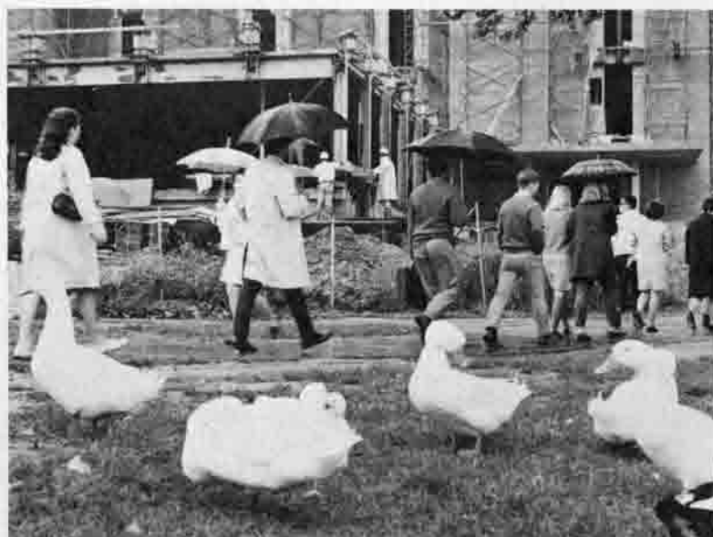
Rain on the first day of school may have dampened the spirits of umbrella-carrying students, but the steady downpour did not bother the ducks resting near the Life Sciences building under construction.
